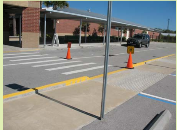
A free standing curb located near the accessible parking spaces may create a trip hazard
