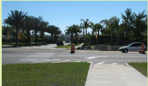
Temporary crosswalk striping does not provide a direct route for students crossing Williamson Boulevard
